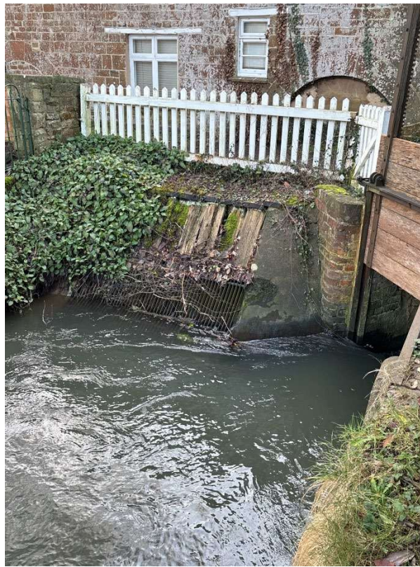
Figure 22 – Disused Mill channel and side sluice diverting flow back into the Sor Brook. (Source: Site visit Jan 2025)
