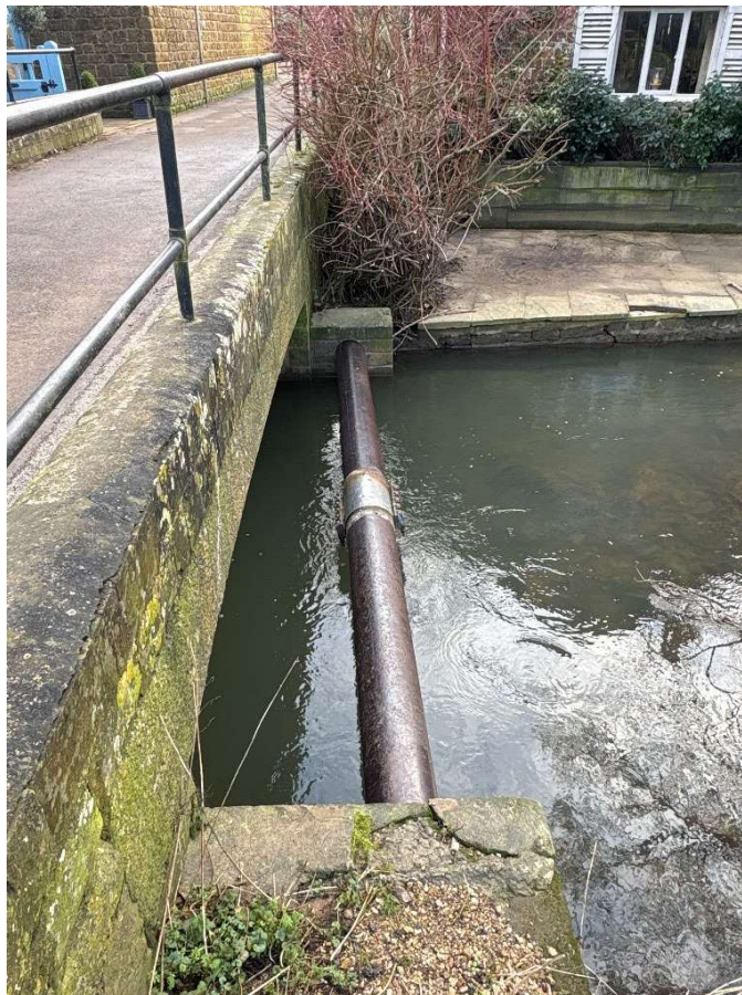
Figure 20 – Thames Water pipe along Sor Brook on downstream side of the Dog Close bridge. (Source: Site visit Jan 2025)
