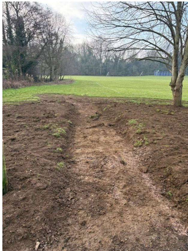
Figure 21 - Slipway being cut along field adjacent to Dog Close to allow water to drain back into the channel more quickly. (Source: Site visit Jan 2025)
